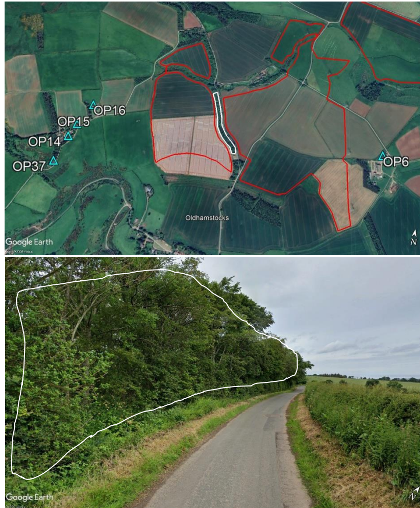
Figure 5-18: Existing screening (white) in between PV arrays 2 & 3 not included in simulation
