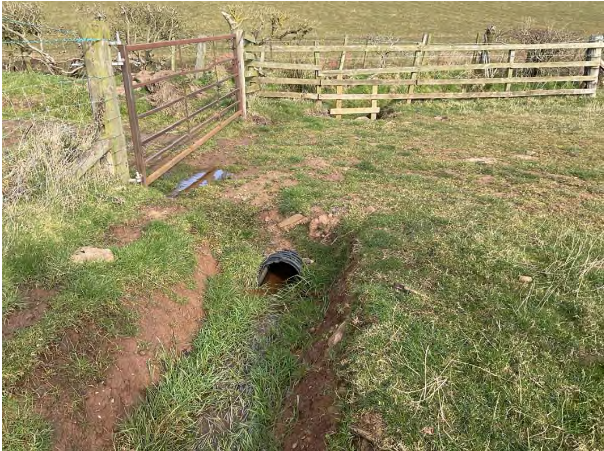
PLATE 6 CULVERT OF A FIELD DRAIN FLOWING INTO TRIBUTARY A
